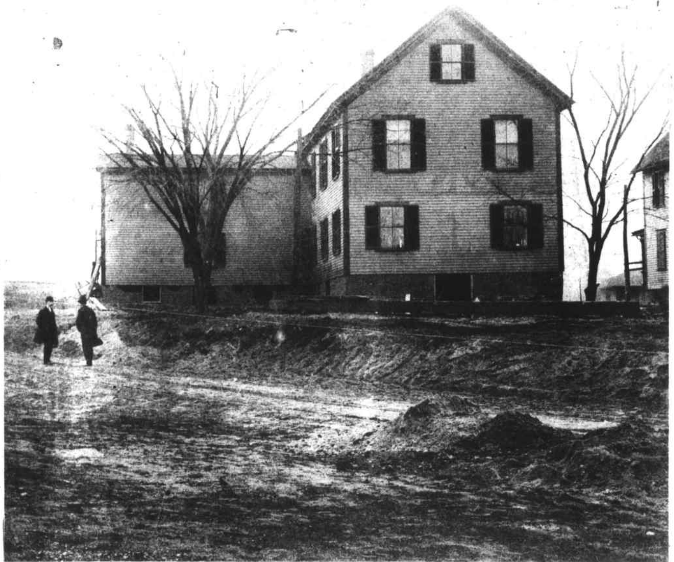
Ames Hall had to be moved, because of the new grade for Church Street. This photo shows it on its new brick foundation, and Church Street being graded. There are marks on the building from contact with a former porch.
